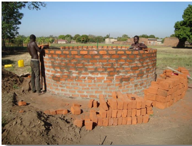
Local Masons building the “Tukul” and Pit Latrine / Bathing facility
