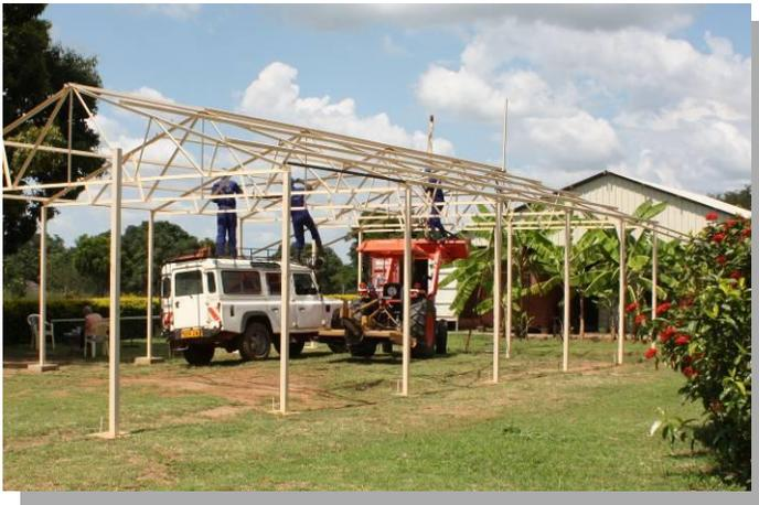
Workmen fitting diagonal bracing to roof trusses a month ago.
