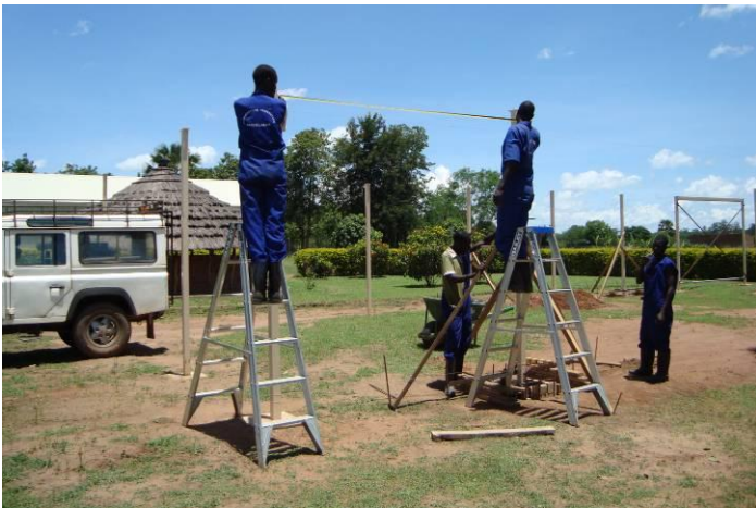
Workmen measuring between posts, while setting up
