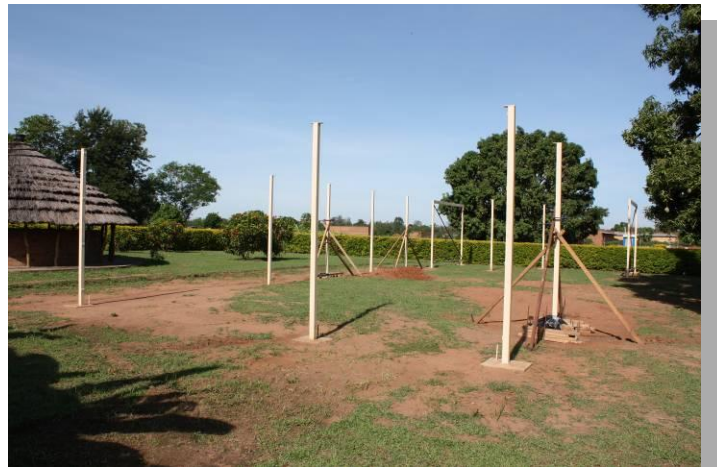
14 of the 24 posts concreted in place
